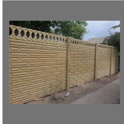
Rcc Compound Wall
