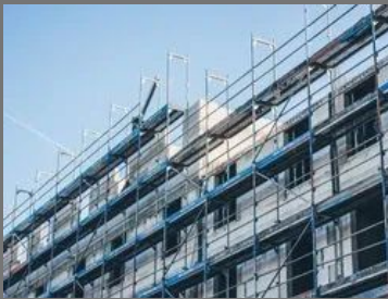
Commercial Building Construction Service
