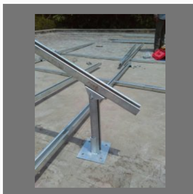
Solar Panel Mounting Structure
