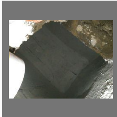
Under Ground Water Tank Waterproofing Services
