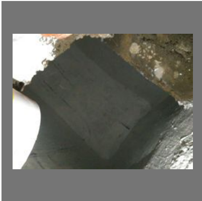
Water Tank Water Proofing Service
