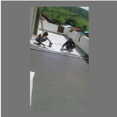
Terrace Waterproofing Coating
