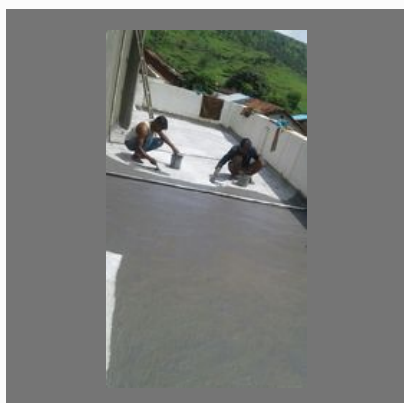
Terrace Water Proofing Services
