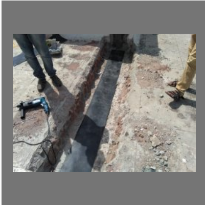
Crack Filling Service
