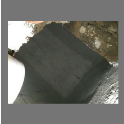
Water Storage Tank Waterproofing Service
