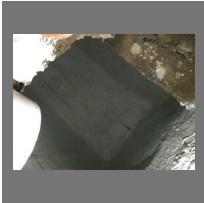
Water Tanks Waterproofing Services
