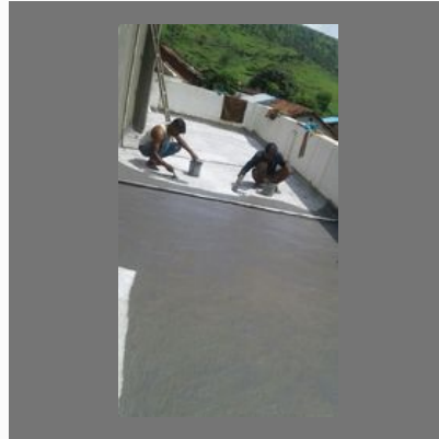
Terrace Surface Area Waterproofing Service
