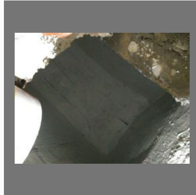
Water Storage Tank Waterproofing Service
