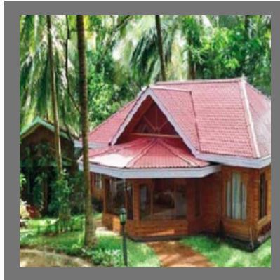
Residential Villas Construction Service
