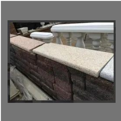
Sandstone Wall Capping
