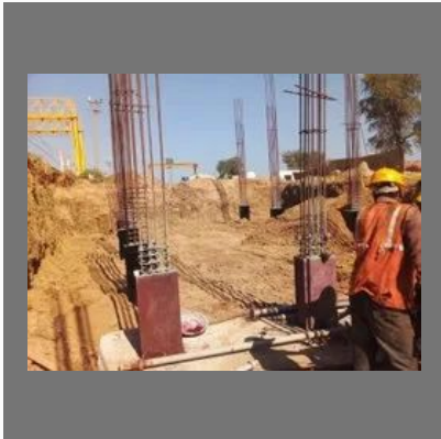
Government Building Construction Service
