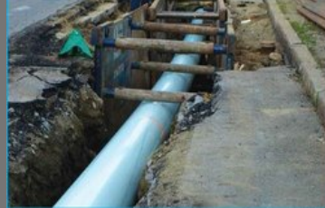
Sewer Pipeline Construction
