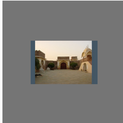
Hotel Nahargarh Construction Service
