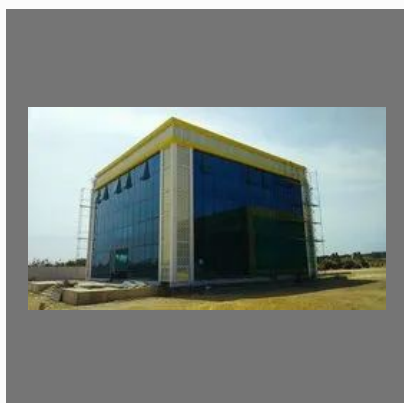
Commercial Building ACP Structural Glazing
