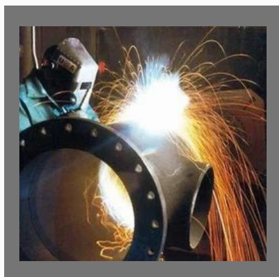
Industrial Fabrication Work
