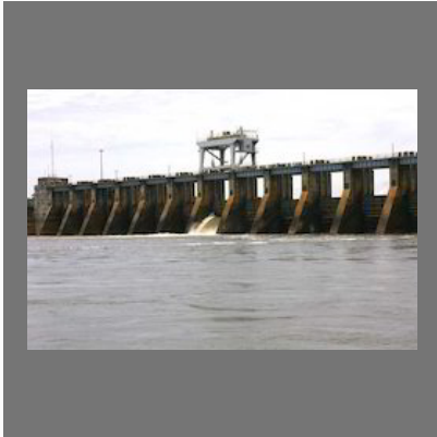
Vertical Dam Gates
