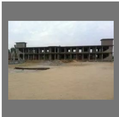
School Building Construction Services
