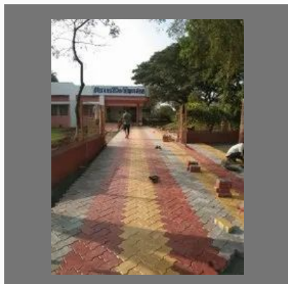
Paver Block Flooring Services
