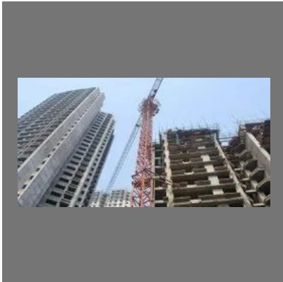
Commercial Buildings Construction Service
