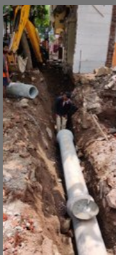
RCC Pipe Work Service
