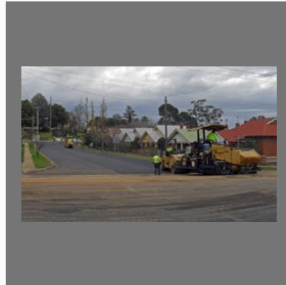
Concrete Road Construction Service
