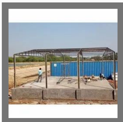
Mild Steel Roofing Structure
