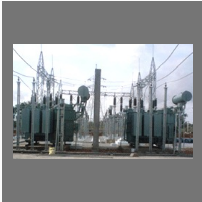
Ehv Sub Stations Construction Towers
