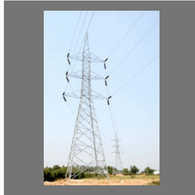
Transmission Lines Construction Towers
