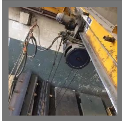
EOT Crane Repairing Services
