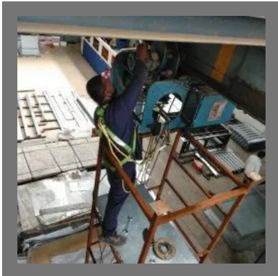
EOT Crane Repair And Maintenance Services
