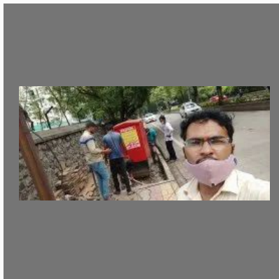
Feeder Pillar Box
