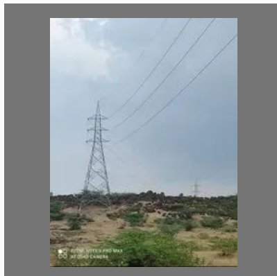
132 KV EHV Tower line Erection
