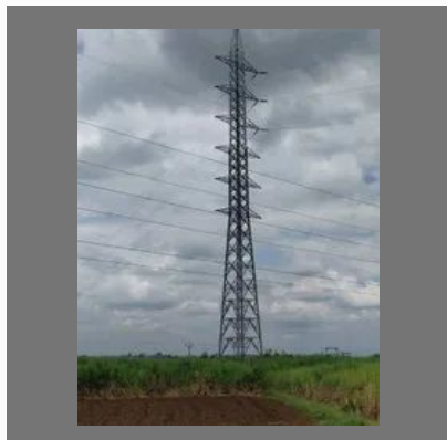
132 Kv EHV Tower Line Erection & Commissioning
