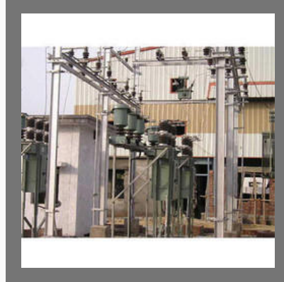
Electrical Turnkey Project
