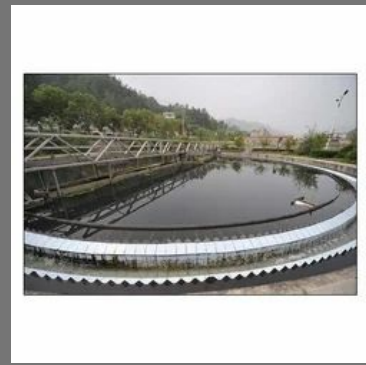
Sewage Water Treatment Plant
