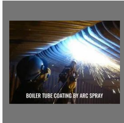
Twin Wire Arc Spray Coating On Boiler Tube
