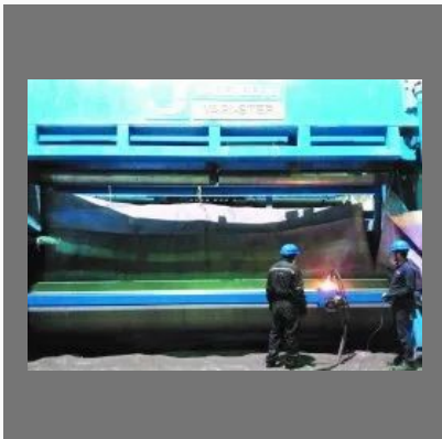
TC Coating On Rewinder Roll
