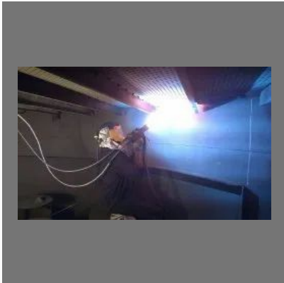
Boiler Tube Coating Service by TWAS Coating service
