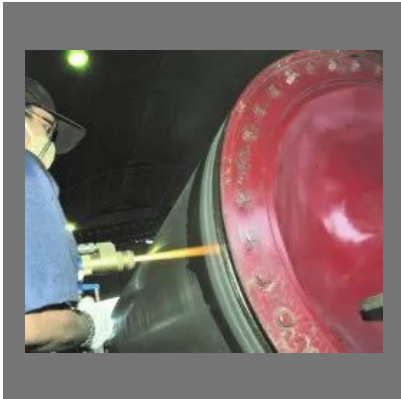
Teflocoat Coating On Dryer Cylinder
