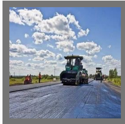
Road Construction Labour Service
