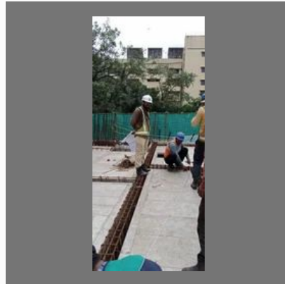
Mivan Shuttering Labour Contractor
