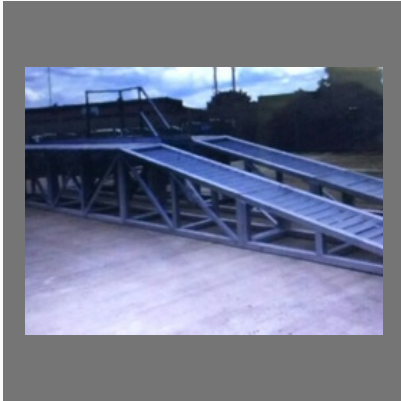
Car Wash Ramp
