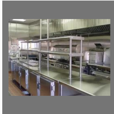
School Canteen Kitchen
