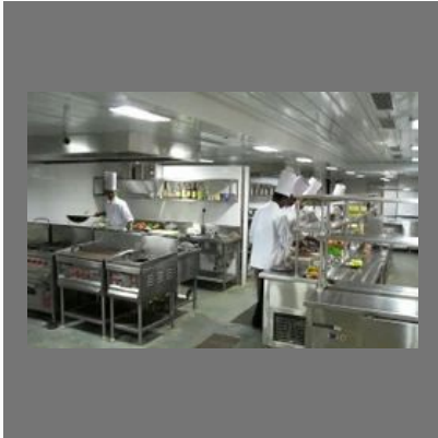
Canteen Kitchen Project Equipment
