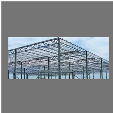
Structural Fabrication Service
