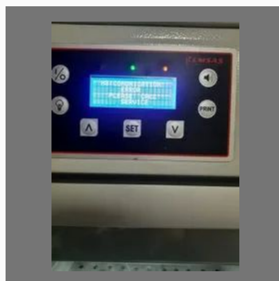
A. C Service. Repair
