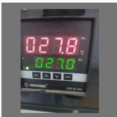
A.c Service. Repairs
