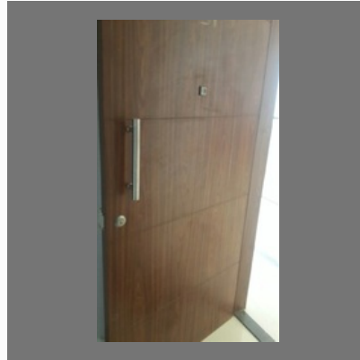
Wooden Main Door
