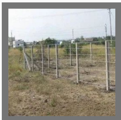
6Feet Rcc Pillar
