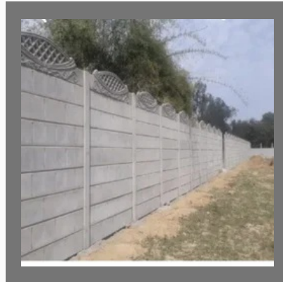
Precast Concrete Walls
