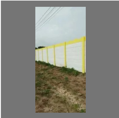
RCC Boundary Wall Compound
