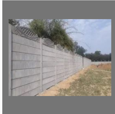
RCC Compound Wall
