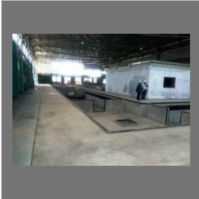
Commercial Buildings Construction Service
