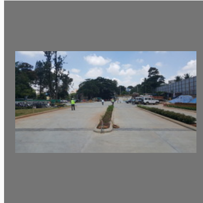
Concrete Roads Construction Service
