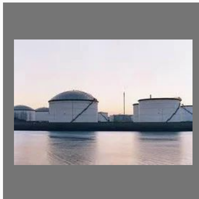
Oil & Gas Industries for Terminal Automation System
