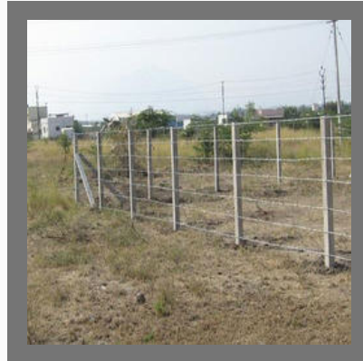
RCC Fencing Work
