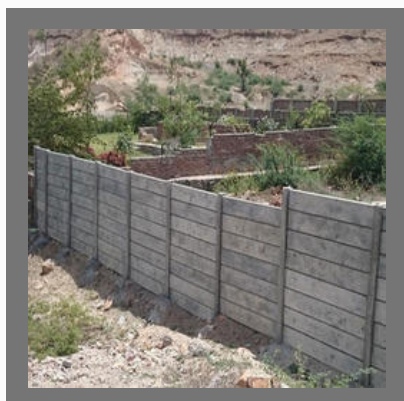
Hollow Block Compound Wall
