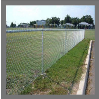
SS Fencing Work
