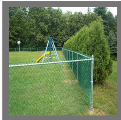
PVC Chain Link Fencing Work
