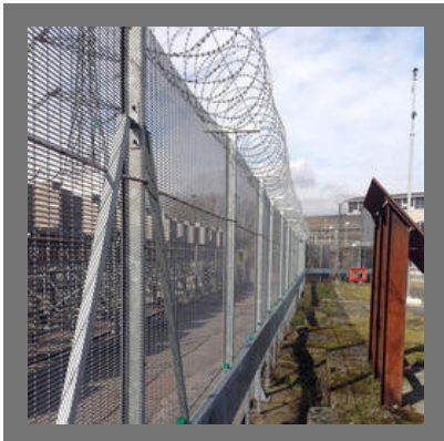
Security Fencing Work
