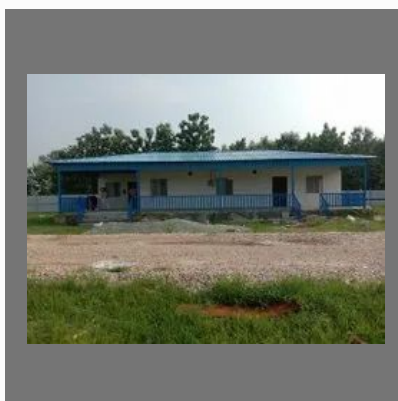
Prefabricated Office Cabin
