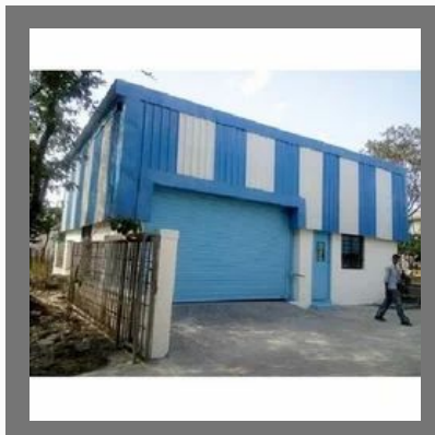
MS Industrial Shed
