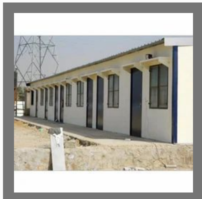
Prefabricated Labour Accommodation
