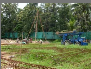
Bridge Construction Services
