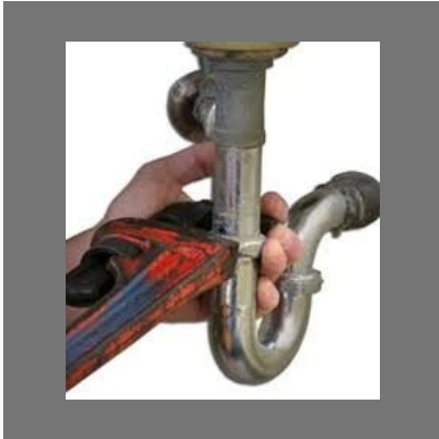
Leak Repair Services
