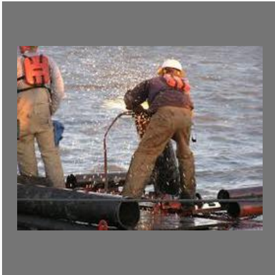
Pipeline Repairs Services
