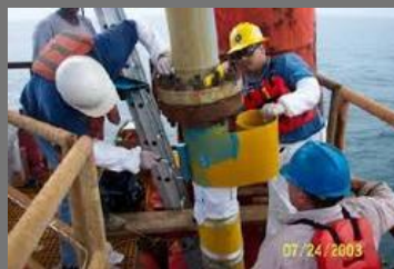
Corrosion Damage Repair Services
