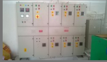
Repair Of AMF And Synchronised Pannel
