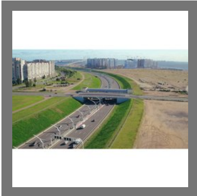
Road Construction Service
