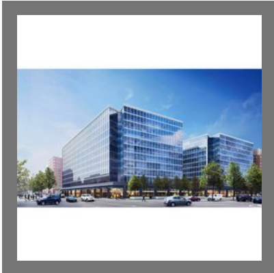
Hospital Construction Service
