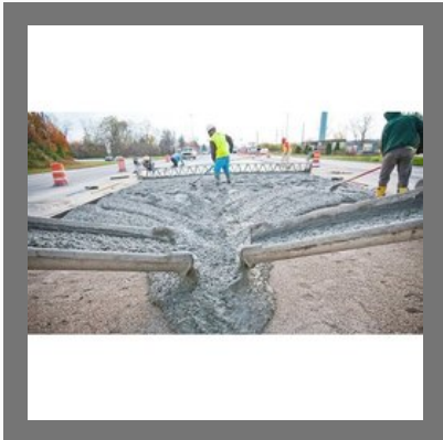
Concrete Road Construction
