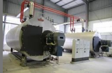
Boiler Water Treatment Chemical
