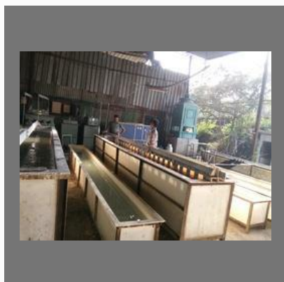
Aluminum Coating Anodizing Plant
