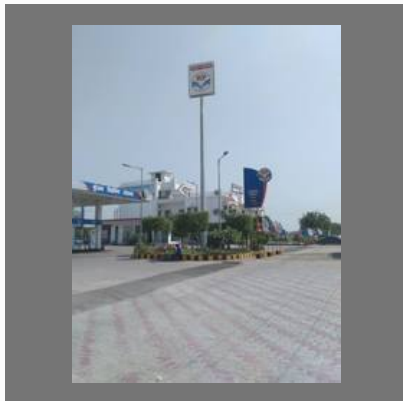
Signage High Mast For Petrol Pumps
