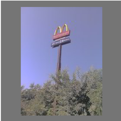
Hoarding Sign Board Installation Services
