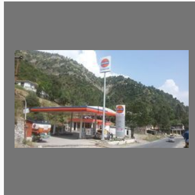
Outdoor High Mast Signage
