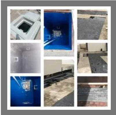
Waterproofing Service and contractors for Water Tank
