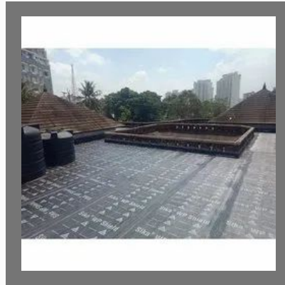
Roof Waterproofing Services
