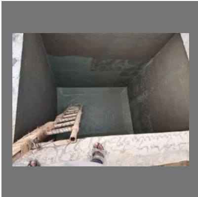
Overhead Water Tank Waterproofing Service
