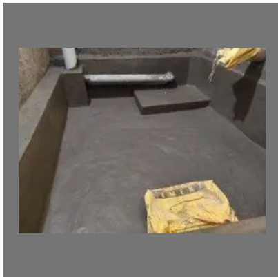
Water proofing Cemntitious Service and contractors
