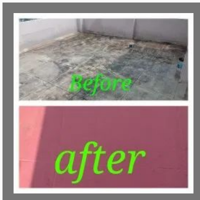
Terrace Waterproofing Treatment Service
