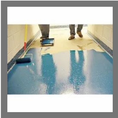
Epoxy Floor Coating Service
