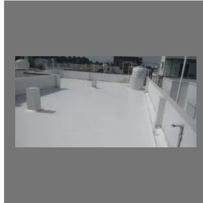
Roofing Waterproofing Service and contractors
