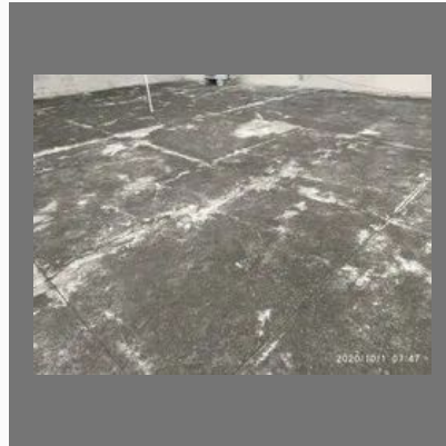
Floor Crack Filling Service
