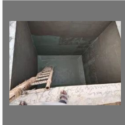
Water proofing contractor for Water Tank
