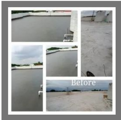
Terrace Waterproofing Treatment Service
