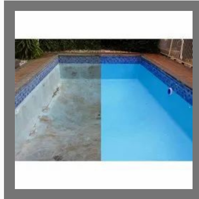
Swimming Pool Epoxy Coating Service
