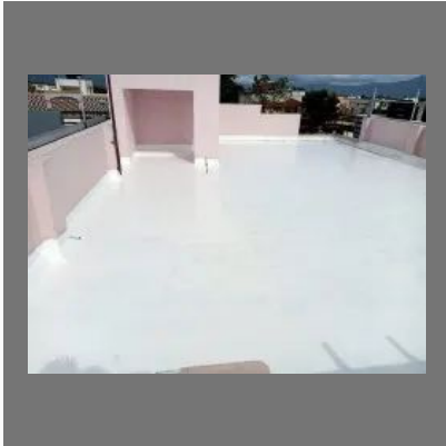
Roof Waterproofing Service
