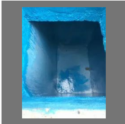
Water Tank Painting Waterproofing Contractors
