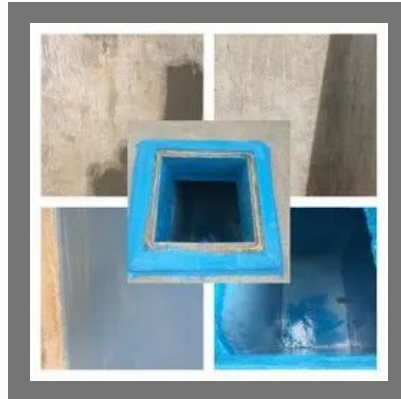
Basement Water Tank waterproofing Services
