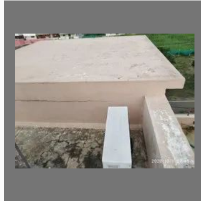
Building Expansion Joints
