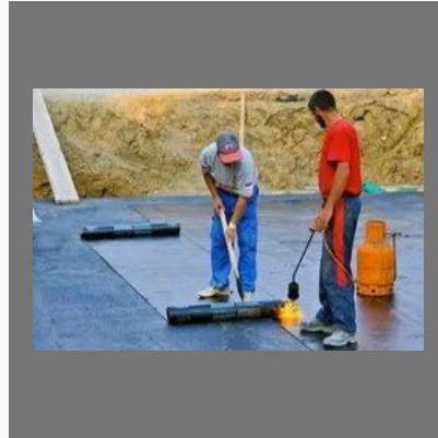
Residential Waterproofing Service
