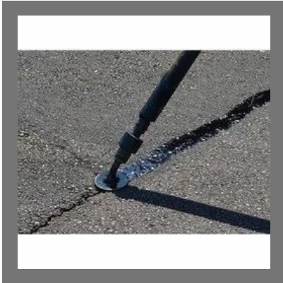
Crack Filling Service
