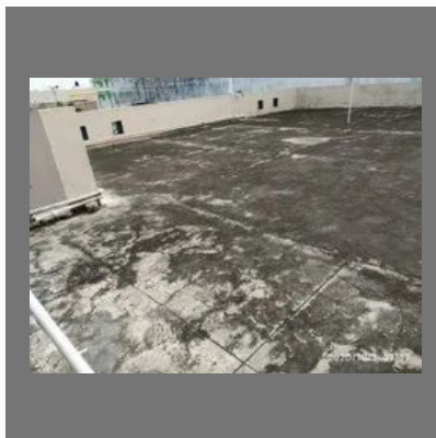
Floor Crack Filling Service
