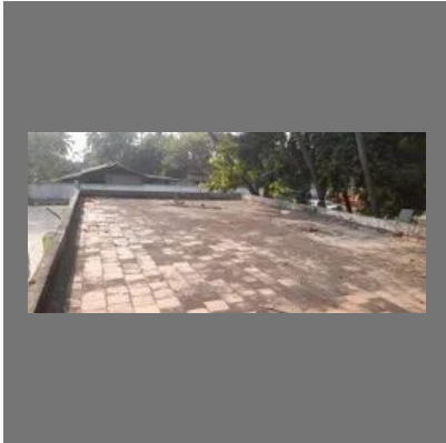
Ceiling waterproofing service
