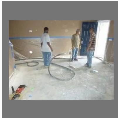
Pressure Grouting Service
