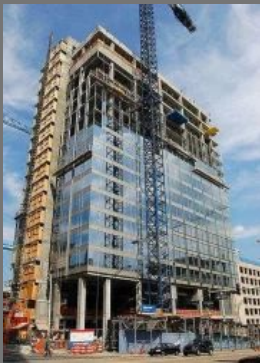
Hotel Construction Service
