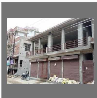
Shop Building Construction Service
