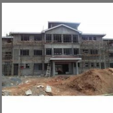
School Building Construction Services
