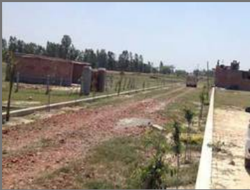
Road Construction Service
