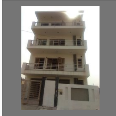
SS Modern Balcony Design
