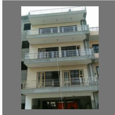
SS Modern Balcony Design
