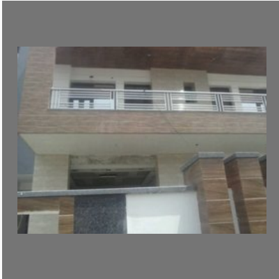
SS Modern Balcony Design
