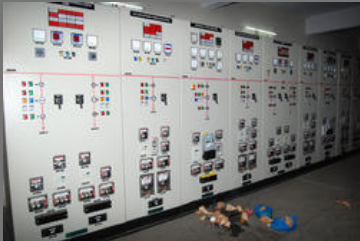
Outdoor & Indoor Substations Works
