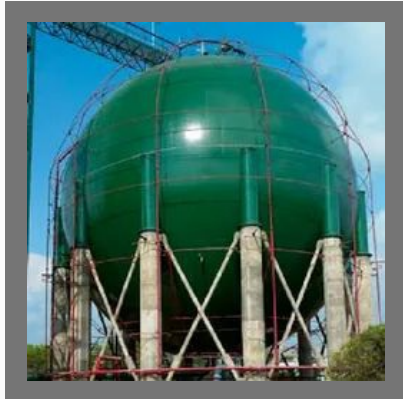
Compressed Natural Gas Service
