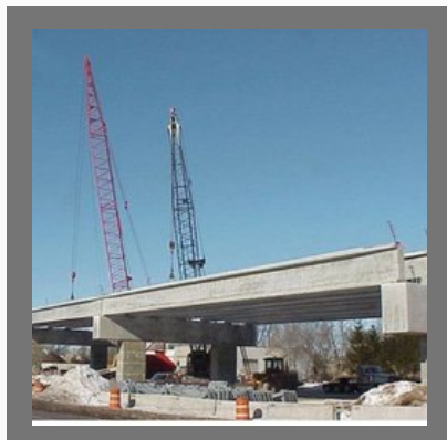
Concrete Bridge Construction Service
