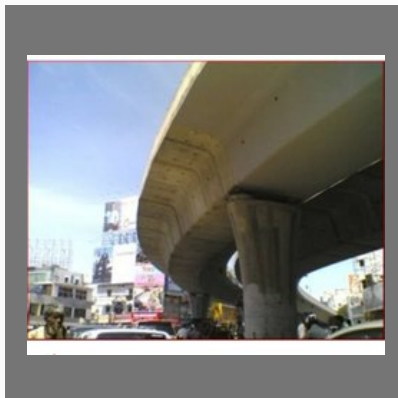
Highway Bridge Construction Service
