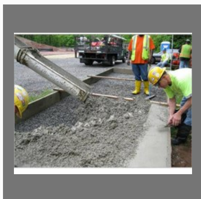
Concrete Road Construction Service
