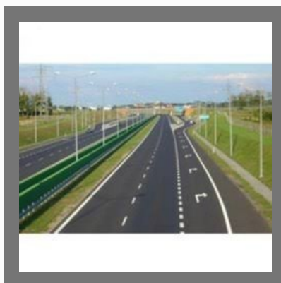
Bitumen Road Construction Service
