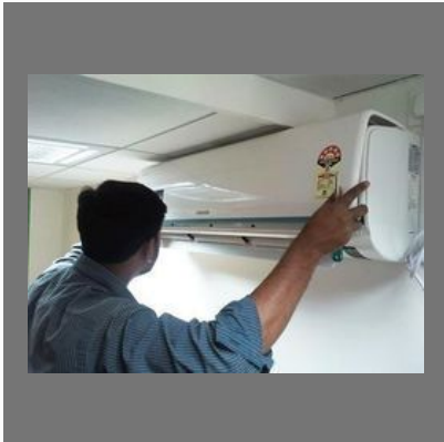
Split Air Conditioner Repairing Services
