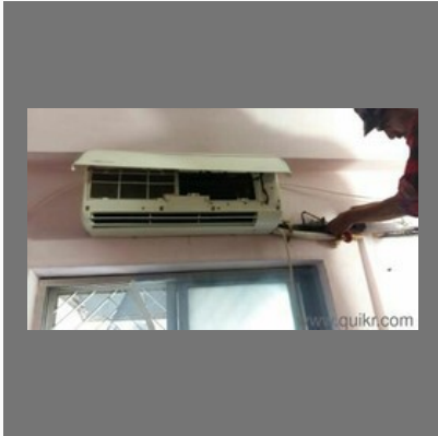
Air Conditioning & Refrigeration Repair
