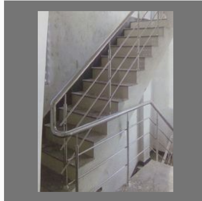
Stainless Steel Railing
