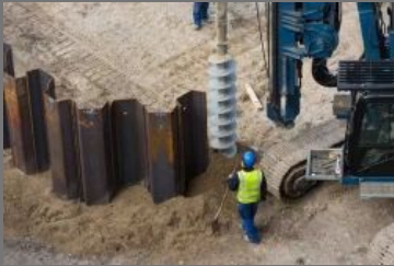
Steel Sheet Piles Foundation Service
