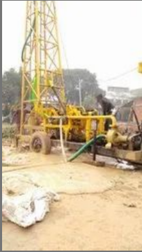
Bored Cast In Situ Piles Services
