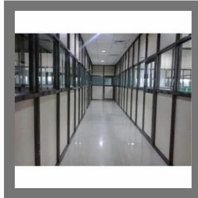
Corridor Aluminium Partition
